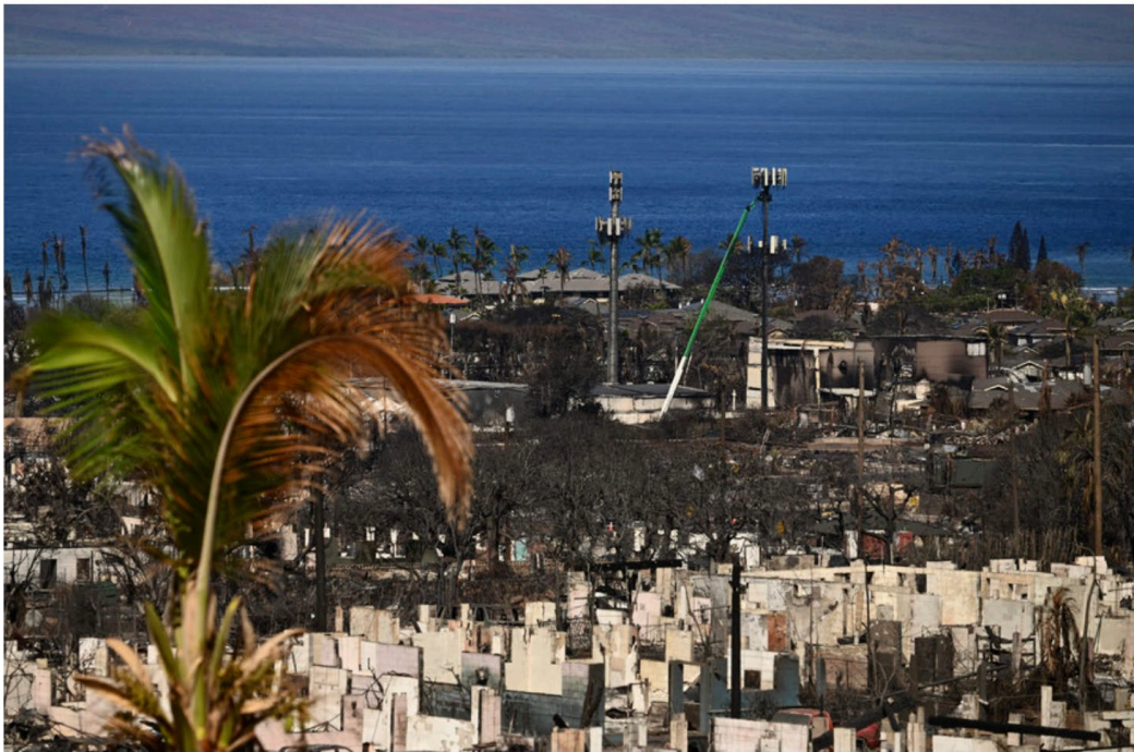
Utility workers repair cellphone service towers in the aftermath of the Maui wildfires in Lahaina, Hawaii, on Aug. 16, 2023. The city and county of Honolulu want the oil industry to pay for spewing greenhouse gas emissions that they say have worsened wildfires and other disasters. | Patrick T. Fallon/AFP/Getty Images
