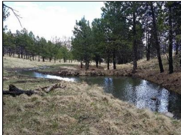
"Plug and Pond" constructed to capture sediment and increase wetland area.
