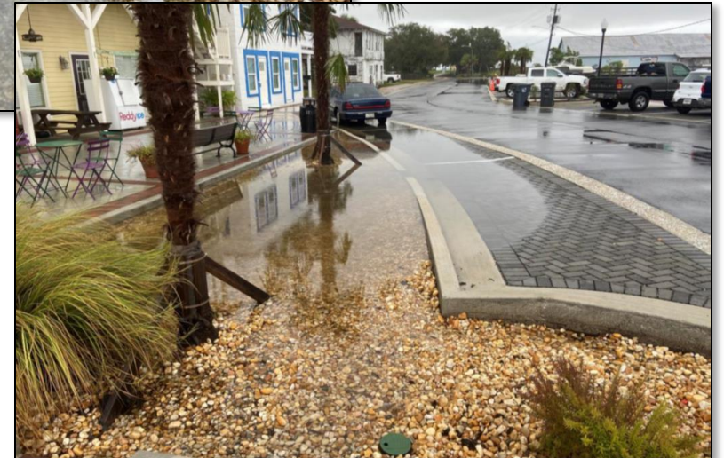
Bioretention system at "Market on Square" reaches capacity & overflows onto permeable pavement
