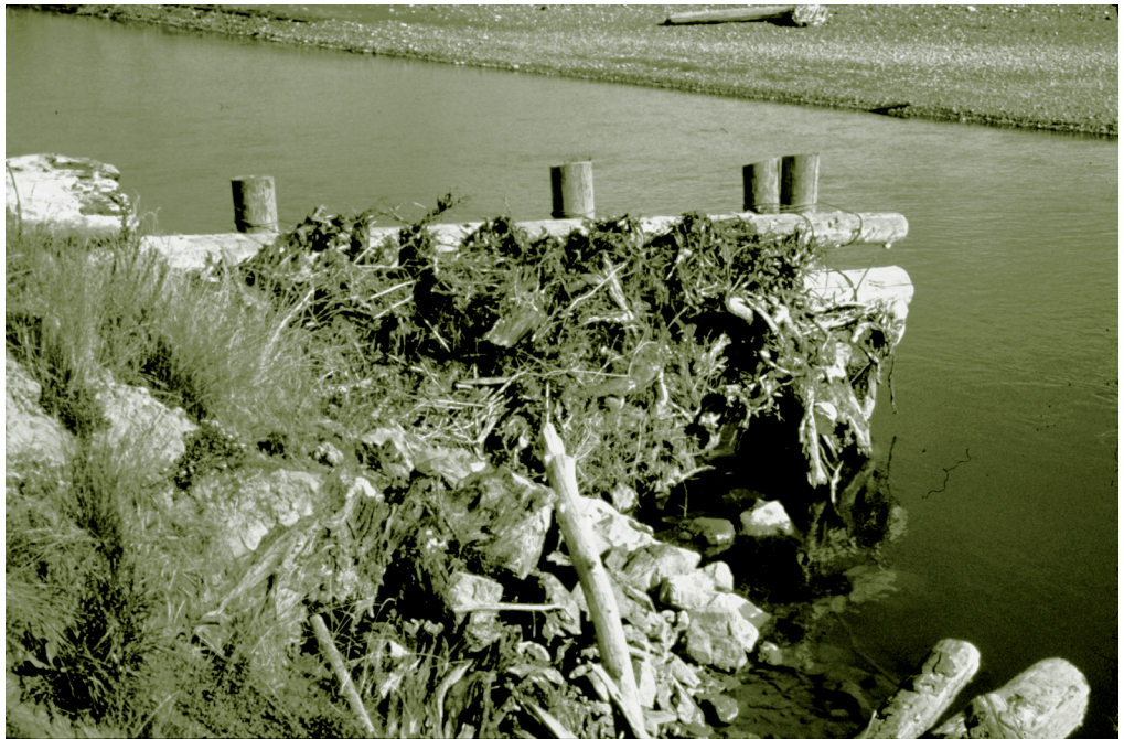
Figure L-4. Woody groins on the Nooksack River.
