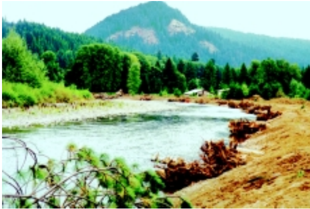
a. Wood Groins with bank reshaping and plantings. During Construction. Wind River. 1999.
