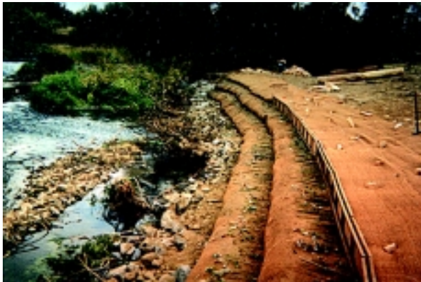
b. Soil Reinforcement lifts with log and rock toe. Salmon Creek, Tributary to Columbia River. 1997.
