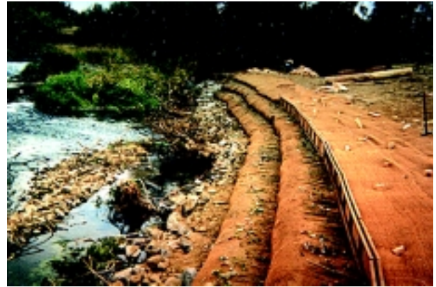
c. Large Woody Debris embedded in Rock Toe. Salmon Creek, Tributary to Columbia River. Source: Inter-Fluve, Inc.
