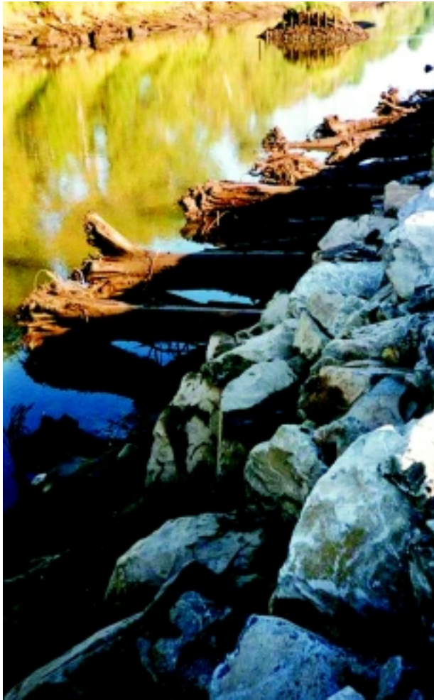
a. Large Woody Debris embedded in Rock Toe. Green River. Source: King County Department of Natural Resources.
