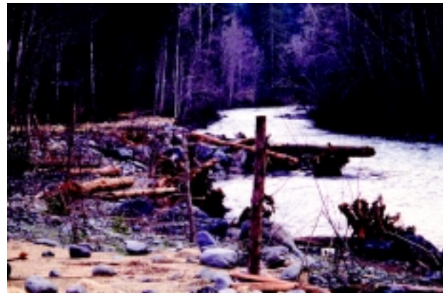
d. Large Woody Debris embedded in Groins. Big Quilcene River. 1997.
