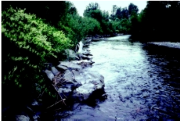
a. Roughened-Rock Toe with reinforced large woody debris and plantings. Cedar River. 1999.
