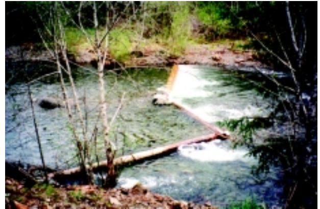
d. Vee Log Drop Structure.
