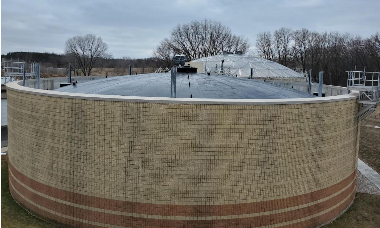
**Figure 3. New 1.5-million-gallon anaerobic digester, converted from a wastewater solids storage tank in 2018.**
