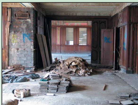
The Skirvin Hotel in Oklahoma City before renovation.
