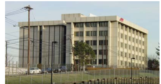
Givaudan site reinvented by the Morris Companies to include three warehouse/distribution buildings totaling 774,000 square feet and the Mountain Development Company (Mountain Technology Center), a modern, high-tech office building of 211,000 square feet, depicted above.
