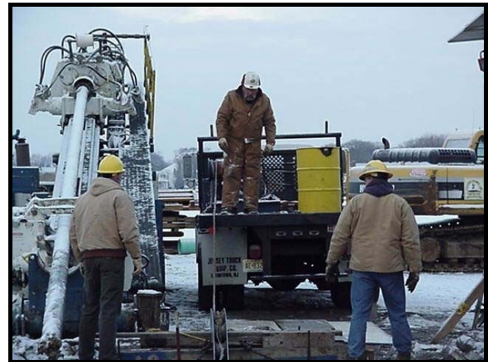
Horizontal Directional Drilling (HDD)
