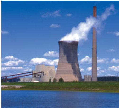
Mountaineer Plant - New Haven, WV
